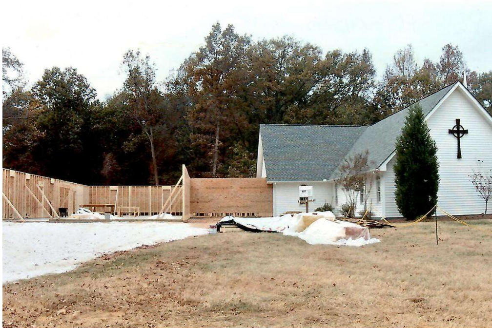
Phase 2 underway – late 2005
