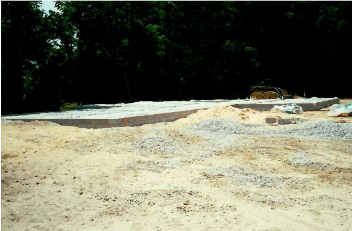
Constructing the slab
